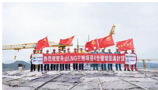
Four new storage tanks of Zhoushan LNG terminal successfully capped
